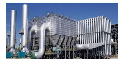
The room-cleaning bag filter has the characteristics of large air volume, compact structure, small floor space, less steel consumption, low energy consumption and convenient operation and maintenance. Dust emission concentration  $\leq$  30mg/m3
